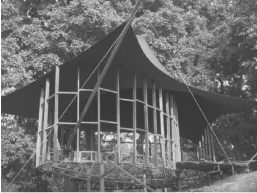
FIGURE 6 Structural system of the tent.
